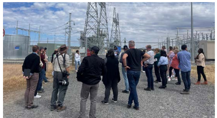
Technical Reference Group members visiting Bulgana Terminal Station
