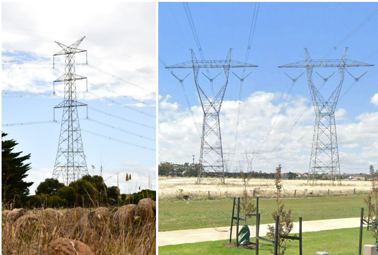
Figure 11.12 500kV double circuit (left); 500kV single circuit (right)
