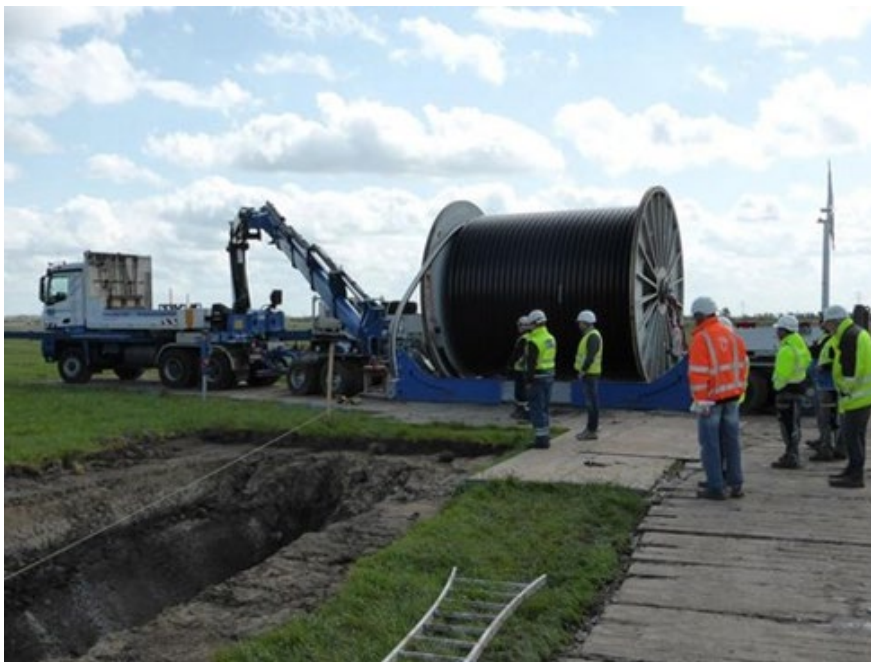
Figure 6 Example of a HVDC cable drum. Source: WWW TenneT Suedlink
