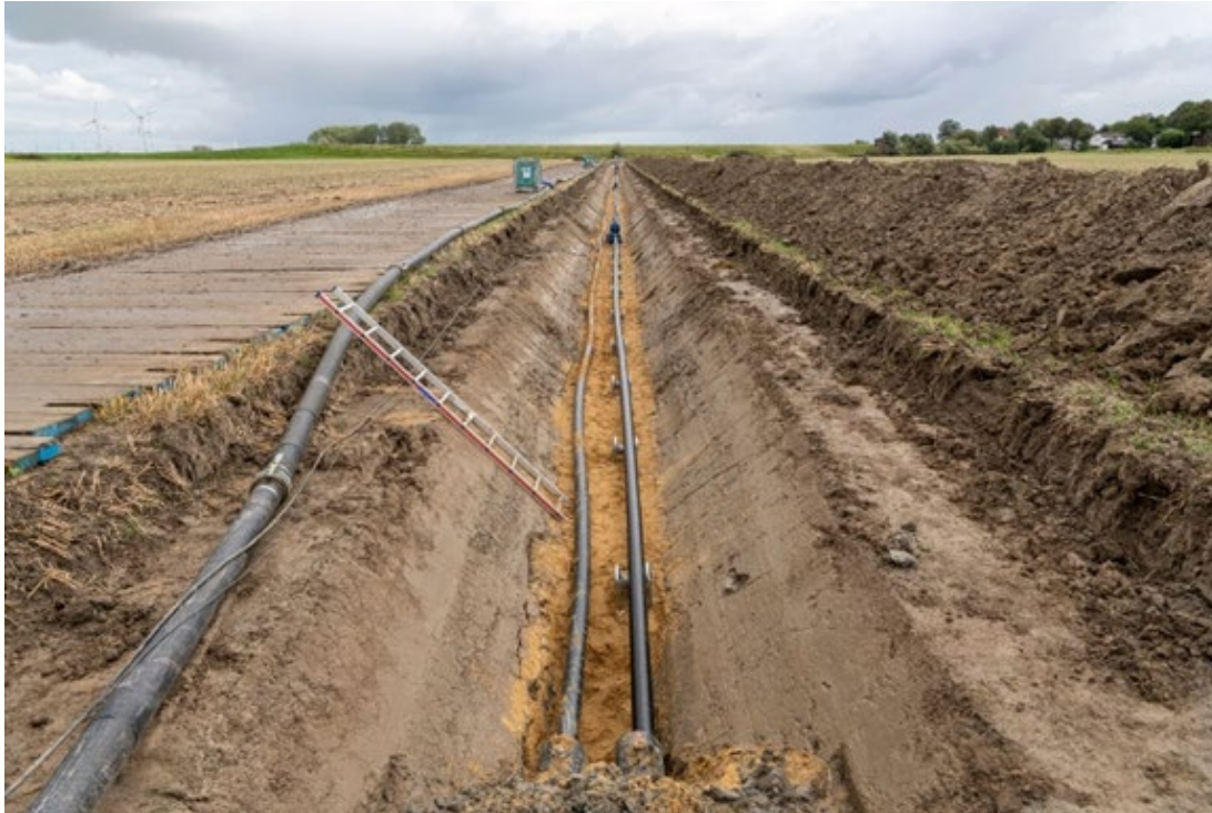
Figure 7 Example of HVDC 525kV cables being laid for SuedLink Source: WWW TenneT Suedlink
