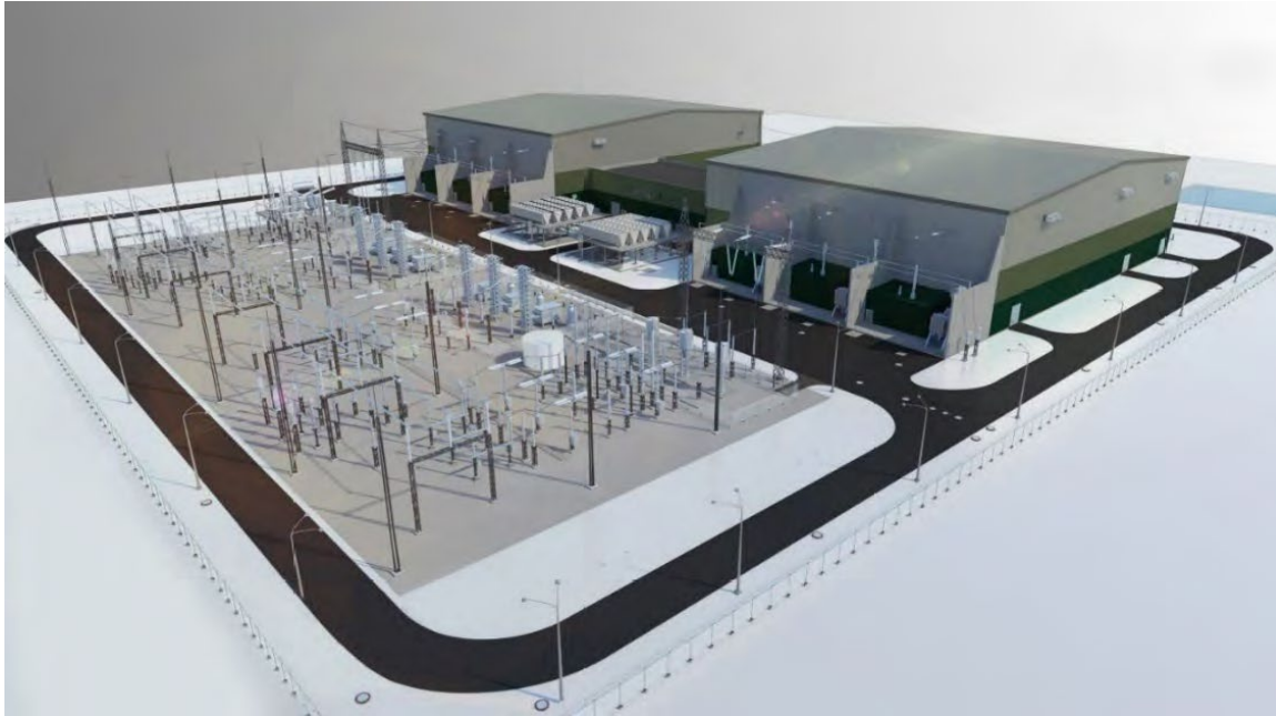
Figure 4 Schematic of Viking Link's Bicker Fen converter station. The facility comprises two voltage source converters. Source: (National Grid UK, 2024)
