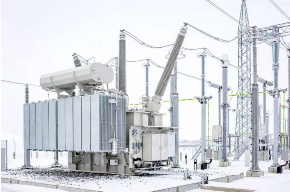
Figure 3 Conceptual image of a typical shunt reactor (type of reactive compensation plant) in a substation. Source: (Hitachi Energy, 2024).
