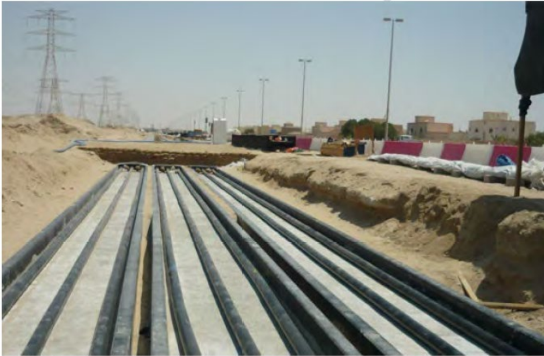
Figure 2 Example of a single circuit 400kV underground cable trench on Sas Al Nakheel to Mussaffah Project
