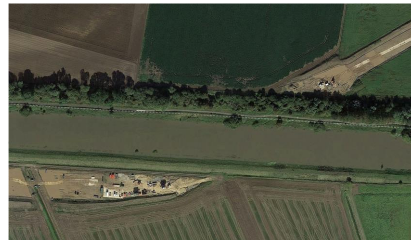
HDD under canal
