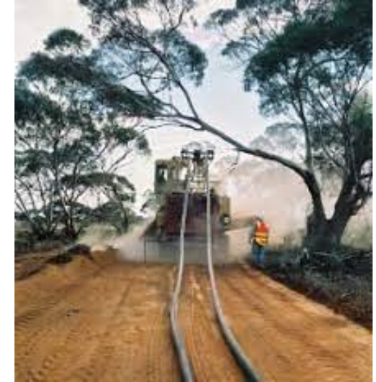
Cable laying (direct burial)
