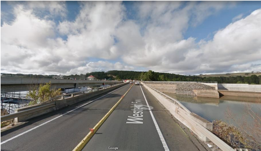
Source: Google Maps (Street view) Image capture 2018 © 2021 Google
