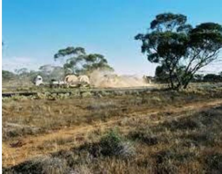
Cable laying equipment
