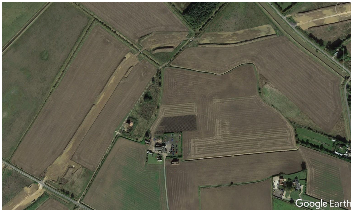
Construction corridor (30 to 50m wide)
