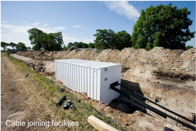
Excavated trench with conduits
