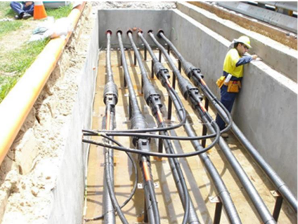
Typical cable joint pit
