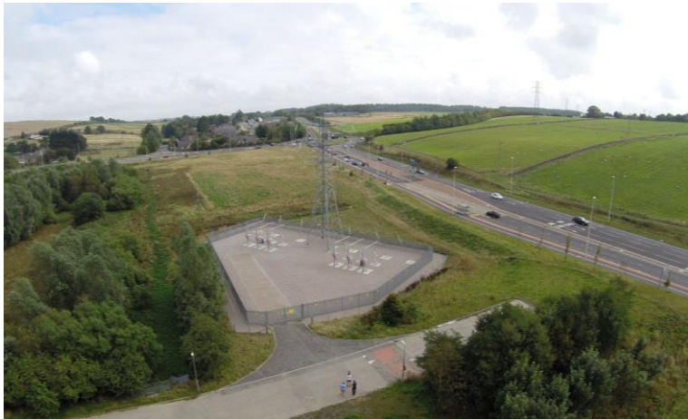
Kingwell transition station Source: Corrie Construction
