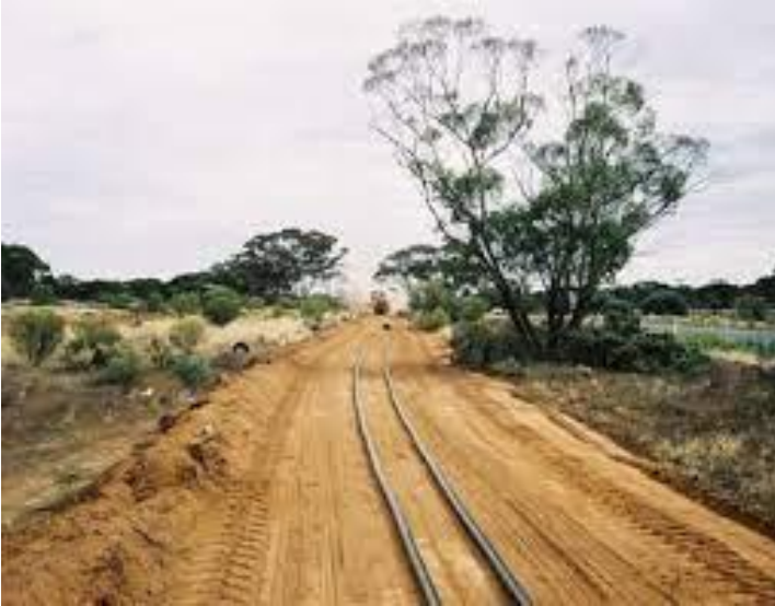
Construction corridor (8 to 10m wide)
