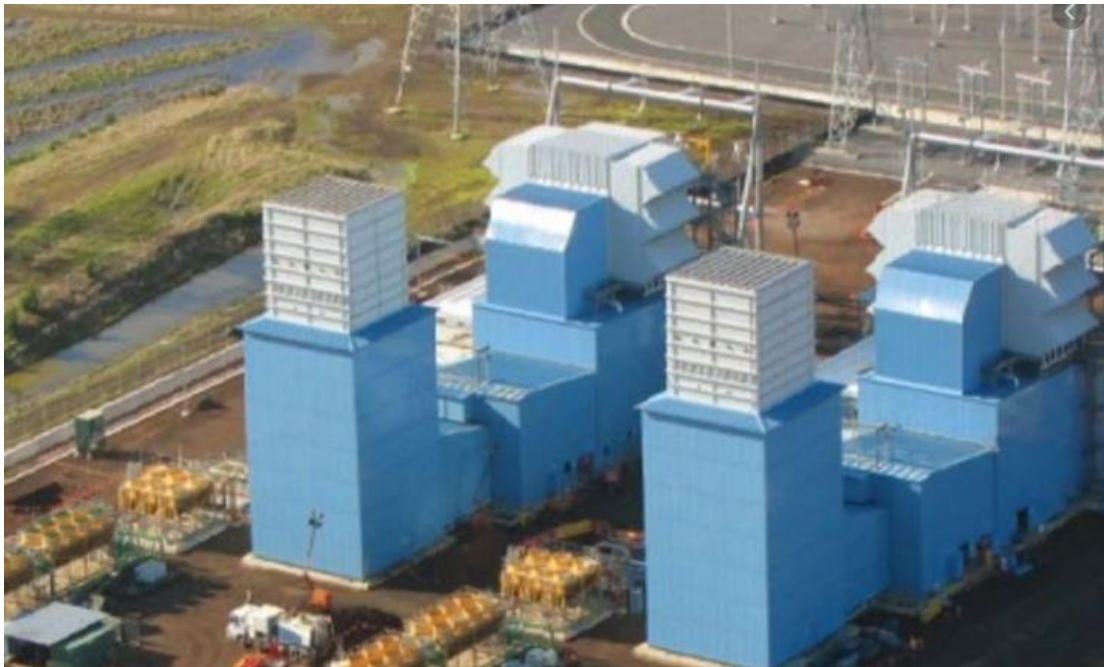
Source: AGL Mortlake Power Station
