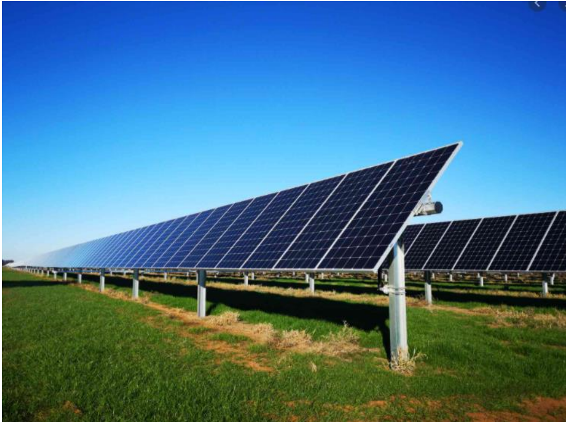
Source: NEOEN Numurkah Solar Farm
