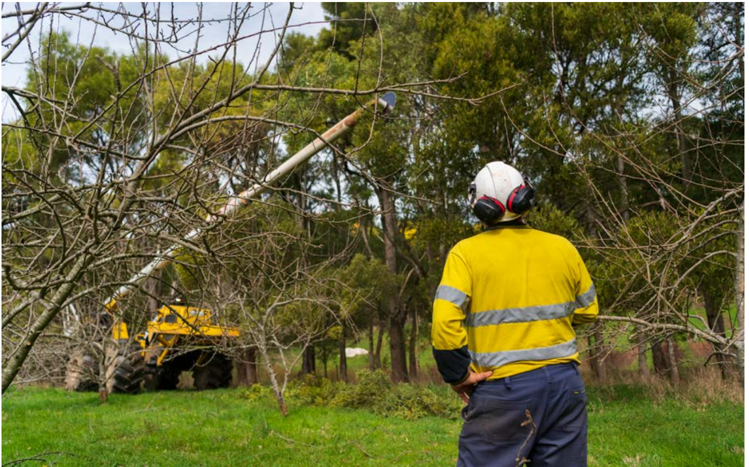
Vegetation may need to be cleared before construction activities begin
