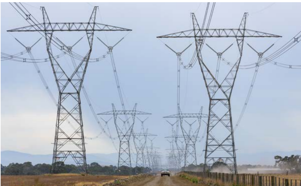
Single circuit transmission towers
