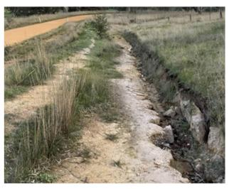
Figure 6.6: Erosion in roadside drain observed near site walkover checkpoint EG-CP07 (Source: Jacobs, 2022)
